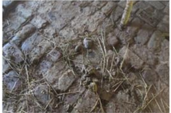
Photo 8. Rough semi-pacca floor of a slaughter house
